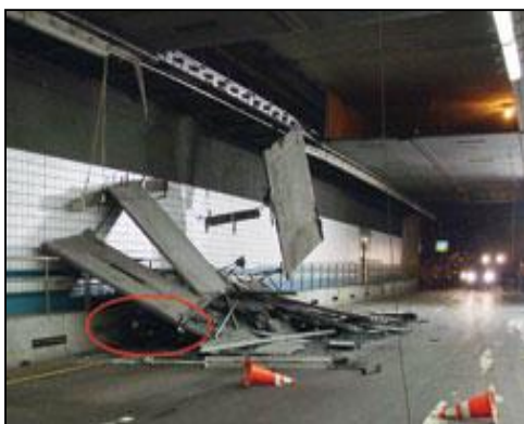
Figure 1 - The ceiling collapse (left) and a simulated view of the cause of the collapse (right)
